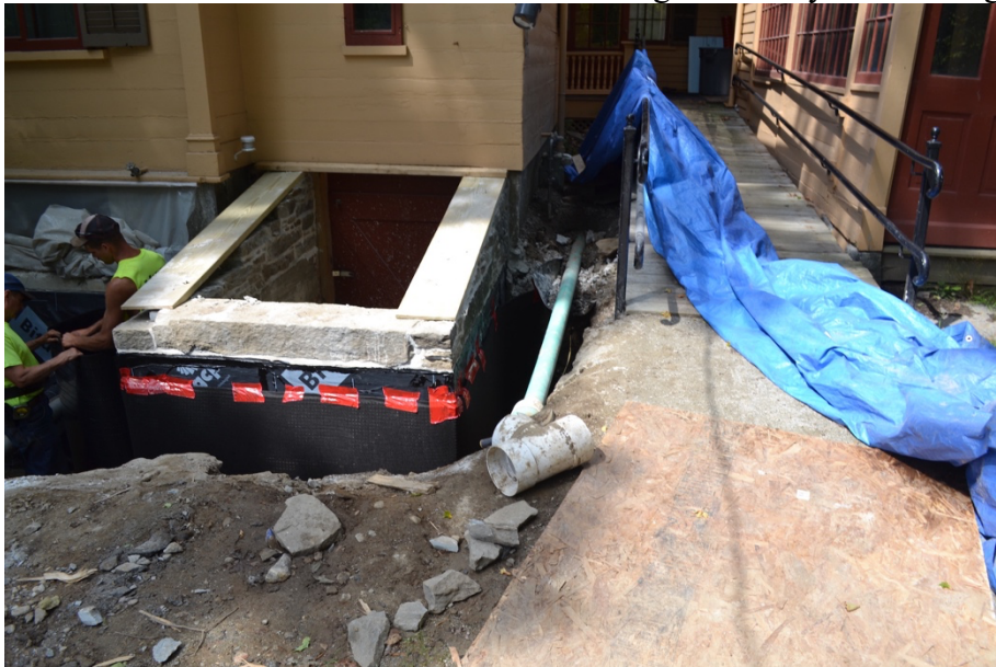
Figure 1: Rebuilt basement bulkhead next to drainage assembly for rebuilt gutter.
